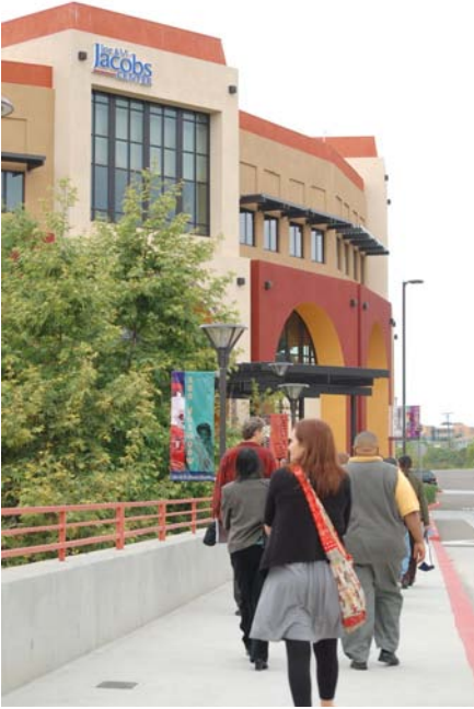
The Joe and Vi Jacobs Center reflects the same vibrant architectural style as the surrounding Market Creek Plaza.
